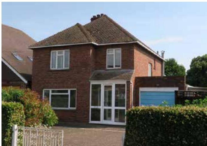
Alex and Stephanie's house prior to retrofitting
